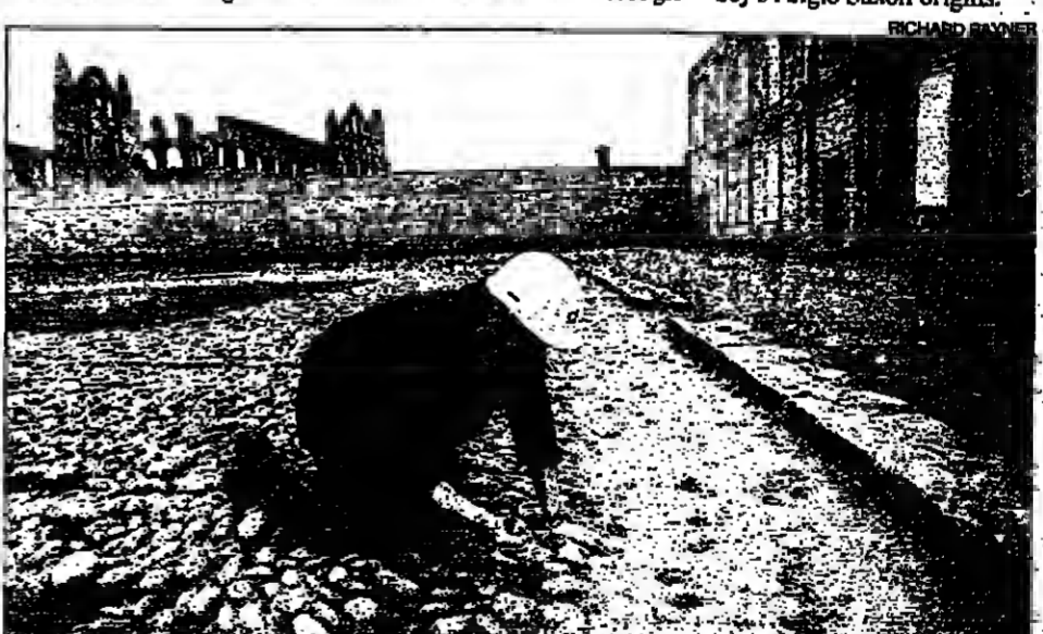
Work begins on restoring the 17th-century stone garden discovered at Whiby Abbey
